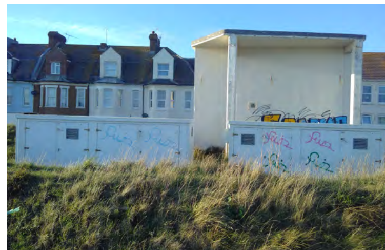
Existing structure on the Bathing Pool site.
